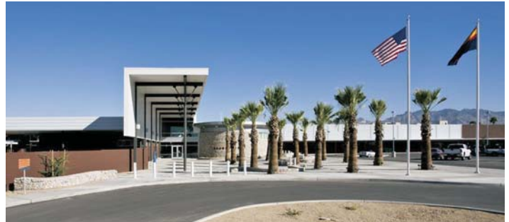
Westside Police Station, Tucson, Arizona A 128,268-sf steel column, steel framed renovation of existing building and added a steel framed auditorium designed by Schneider & Associates
